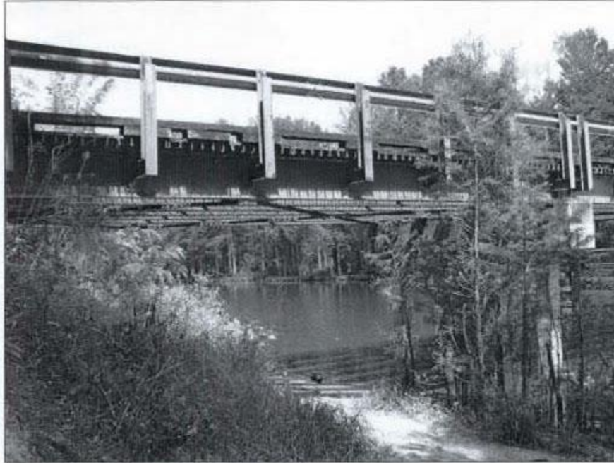
Photograph 4 Roll 2702-1, Exp. 4; Approach Span, Facing North
