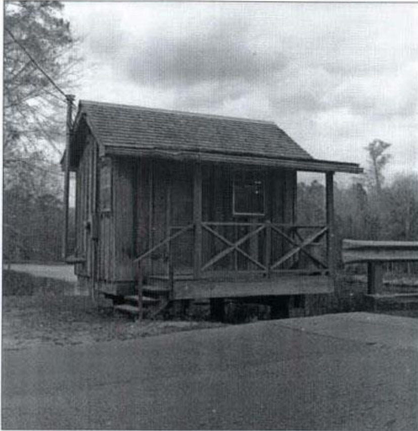
Photograph 11 Bridge Tender's Station, Facing North, 1981 Photograph courtesy of Florida Photographic Collection
