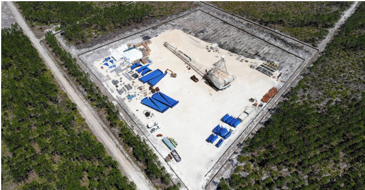
TPM broke ground on staging areas before obtaining required permits. (© Joseph Kelly, Georgia River Network)
